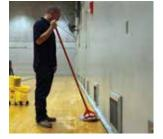
Rinse the floor thoroughly using WAXIE Ultra Clean Wood Floor Cleaner (#320895) diluted at 2 ounces per gallon of water (1:64) in an autoscrubber with red pads, SPP Pads or rinse with a well wrung mop. Mop rinse all corners and edges to insure that the entire floor is rinsed.
