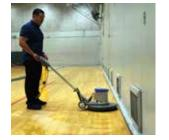
Scrub the floor with a floor machine equipped with maroon colored Surface Preparation Pads (SPP) or 220 grit sand screens. Heel the machine gently on stubborn marks.
